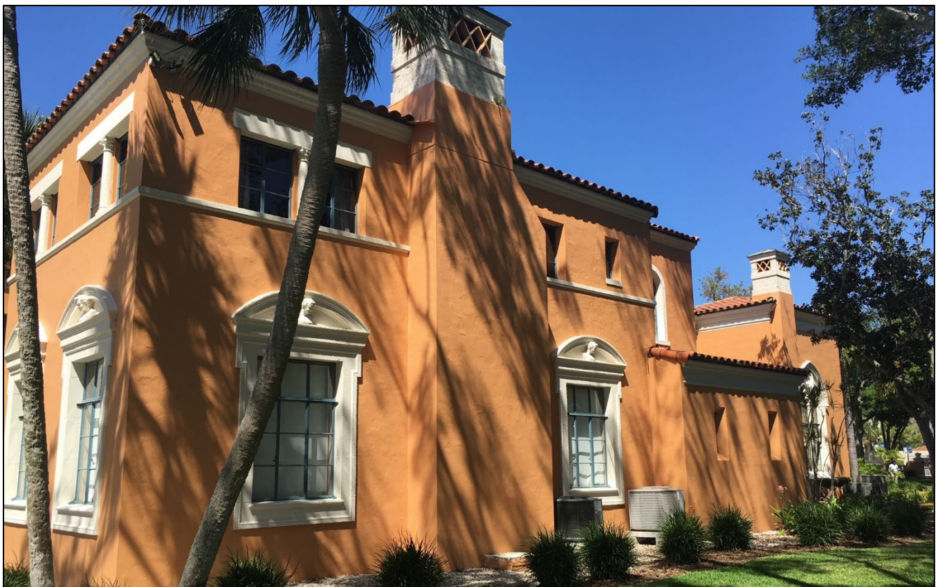
Figure 6: Photograph showing the chimney where the breezeway connection will be attached.
