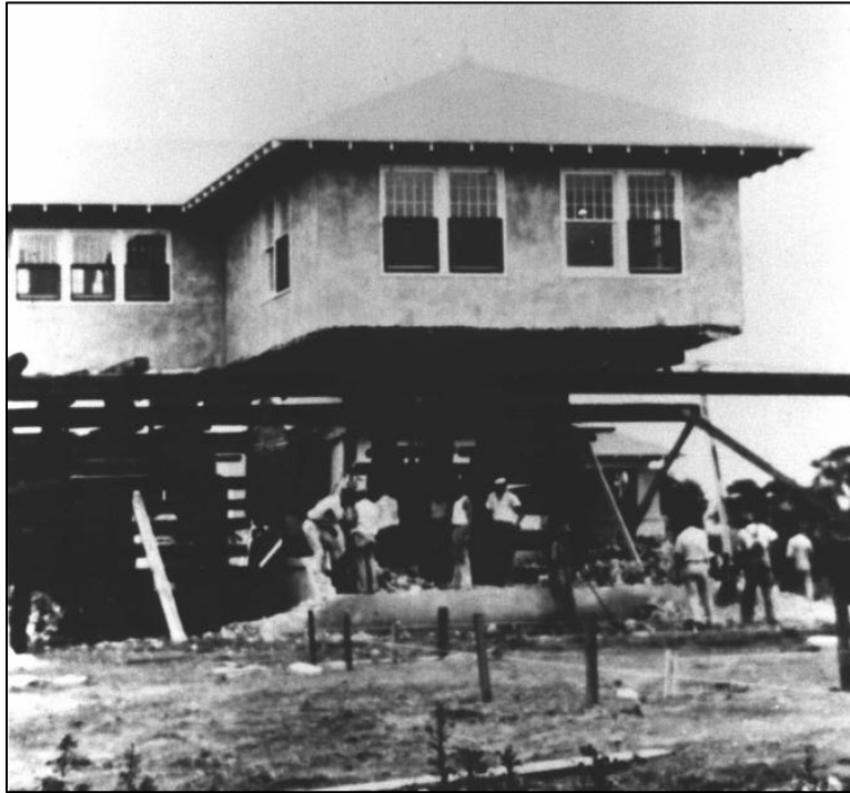
Figure 2: Historic photograph of Casa Coe da Sol under construction. The frame house that was previously on the site was lifted and incorporated into the new construction.
